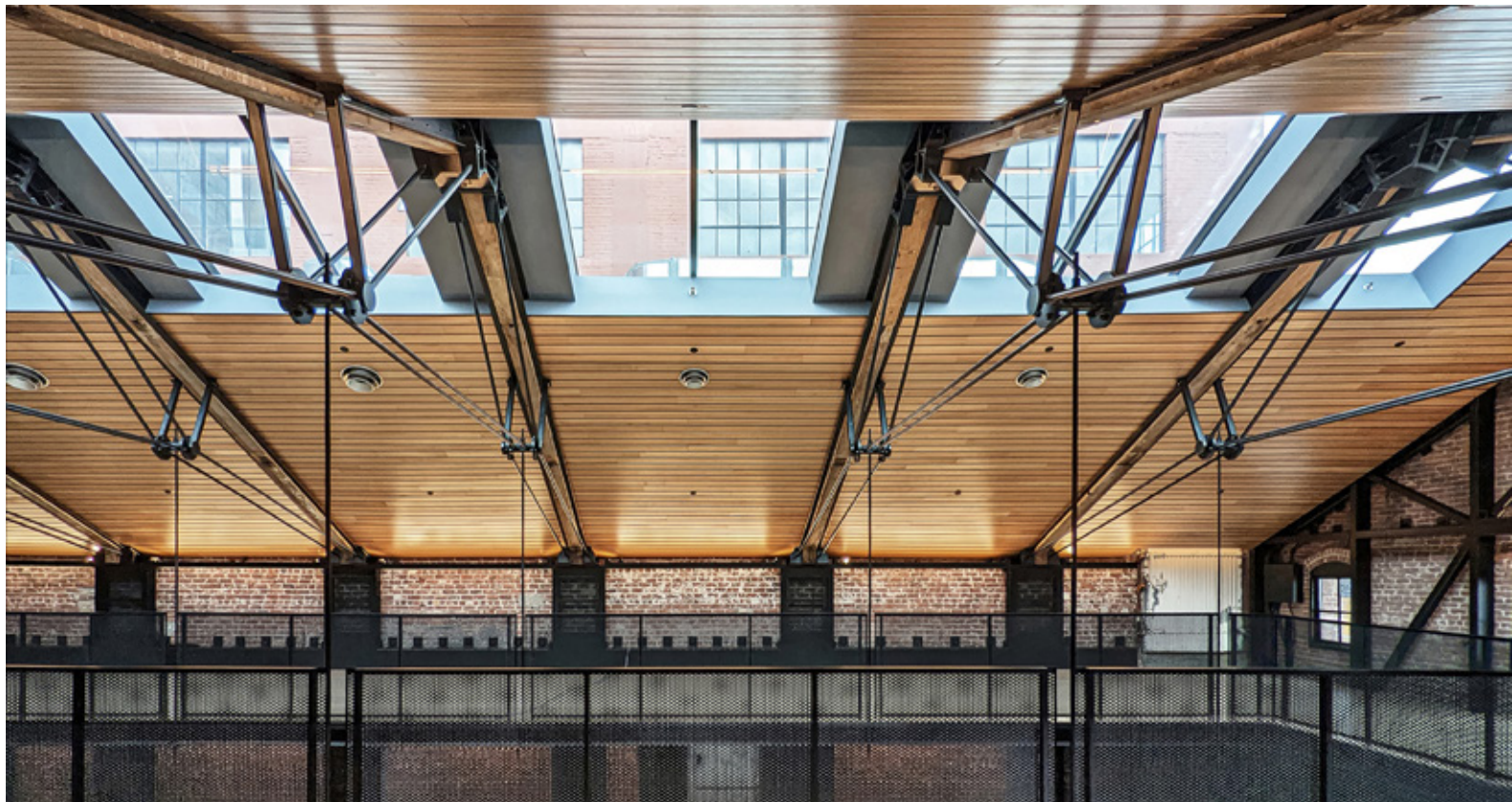
After : Looking South from Mezzanine Photo © Architect
